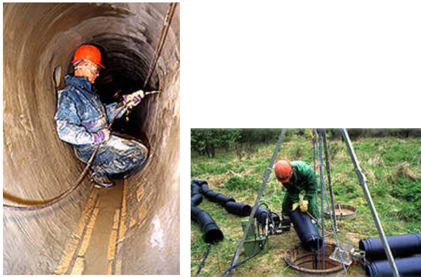
Fig. 4 - 9 Repair and refurbishment of a reach (section of sewer)
