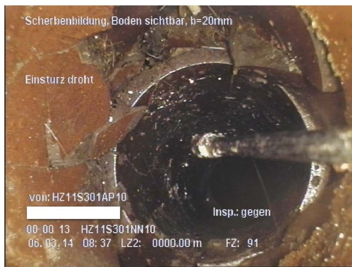
Fig. 4 - 7 Damage in a stormwater sewer with immediate action required
